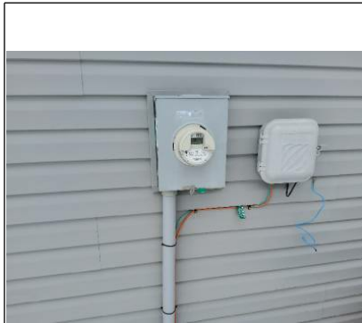
Main electrical service meter.
