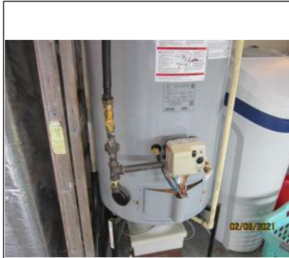
Water heater & soft water tank.
