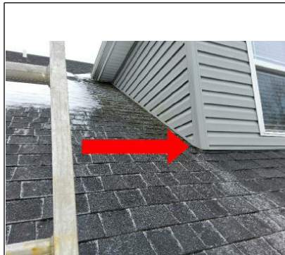
Can not verify step flashing existence.
