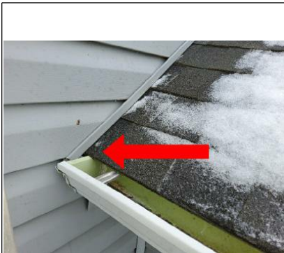
Missing kick out flashing.
