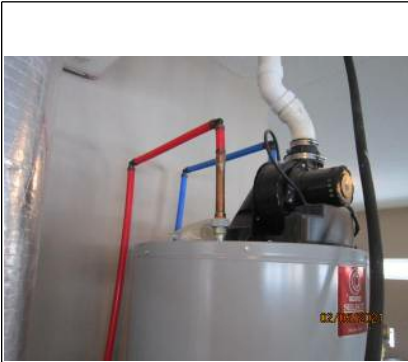
Water heater power exhaust
